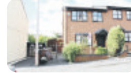
Fidler Street Toll Bar
